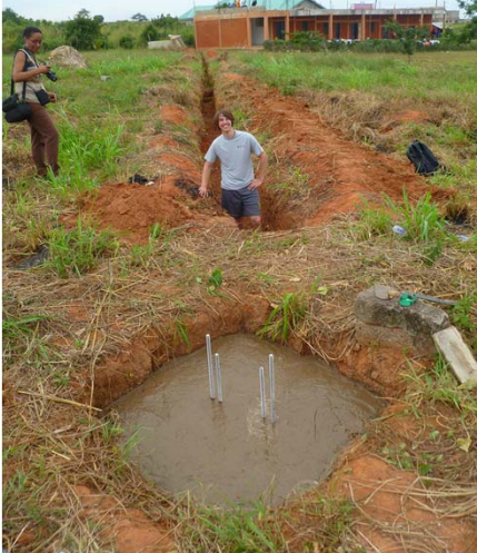
Prof. Rouse and David Newill-Smith '14 await the setting concrete before laying electrical conduit to the school where the charge controller, battery bank and inverter are located.
